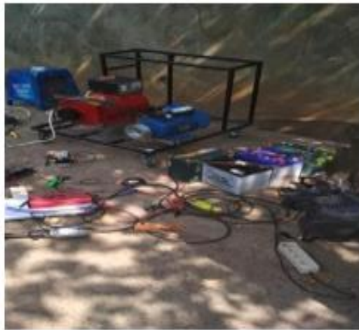
Gambar 5 proses wearing generator set aki ( batere )
